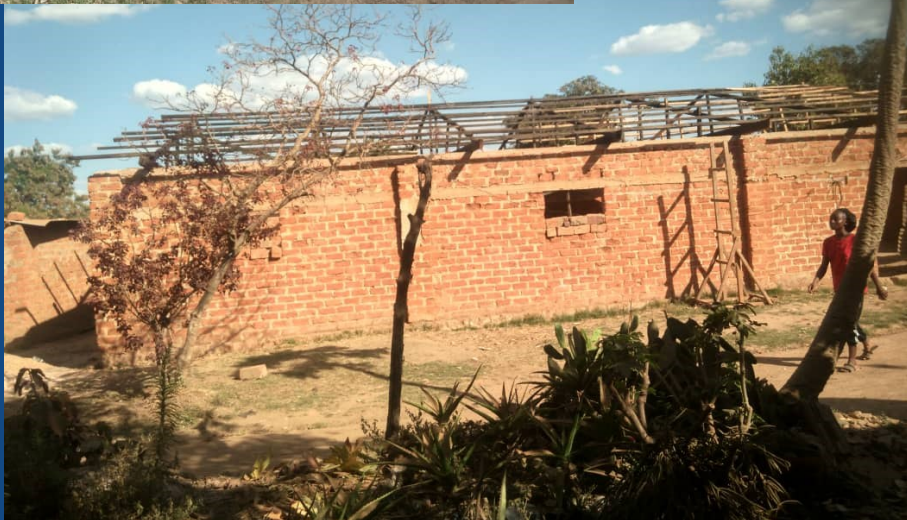
The Matendo Church as progress on the roof continues in June
