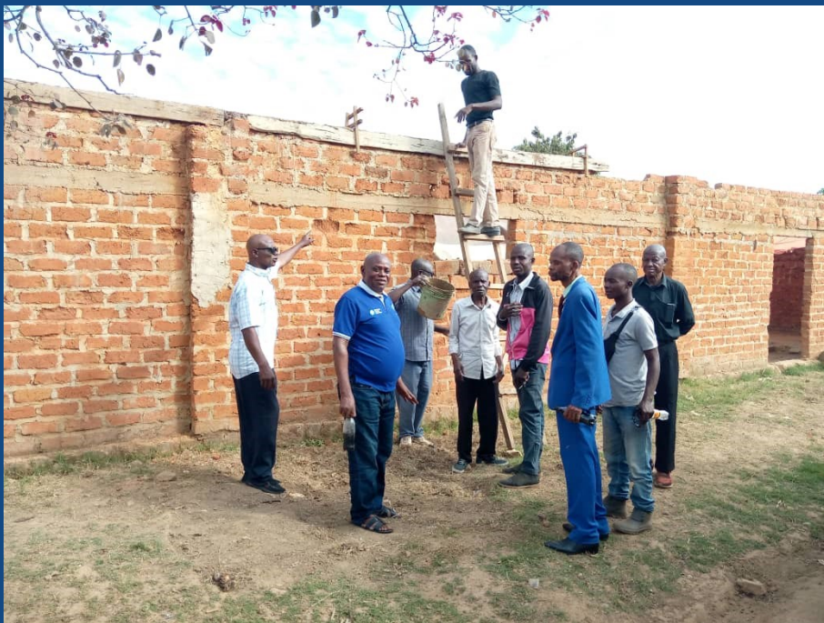
Rev. Cimbanga (second from left) and other church elders inspect the progress on the CEM's Matendo Church in May
